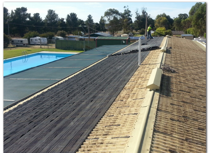
Removing old rubber strip collectors.
